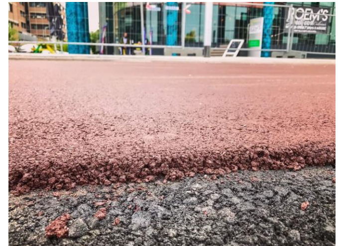
Dutch Cycling Embassy, 2021: 3-cm layer of tinted red asphalt
